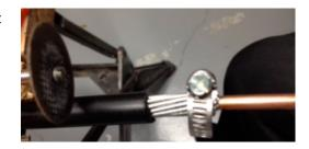
The cable has a hard jack and a torch or heat gun will help for the jacket removal. You will probably remove 6 or 7 feet of outer jacket
